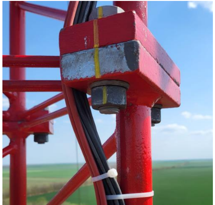
Marked screws on the windmast
