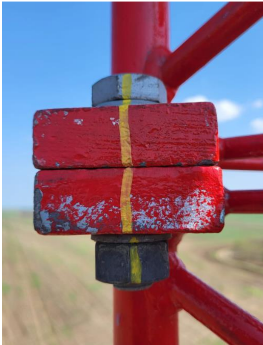
Marked screws on the windmast
